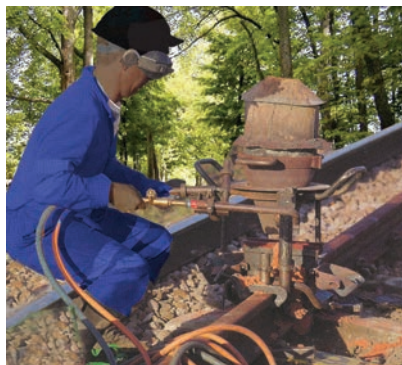
Figure 3.11 Thermit process for joining railway tracks
